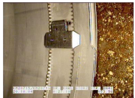
Packer in the middle Application pressure
